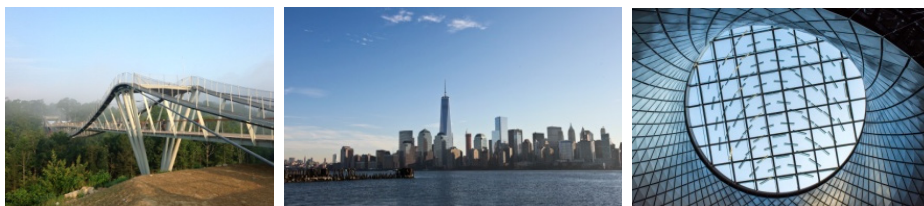
Consol Energy Wingtip Bridge, Skyline of New York with the One World Trade Center, Sky Reflector of Fulton Centre; all: © schlaich bergemann partner
