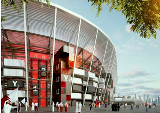
The facade is characterized by the unique container structure, which serves individual functions such as stalls or sanitary fittings. © Fenwick Iribarren Architects
