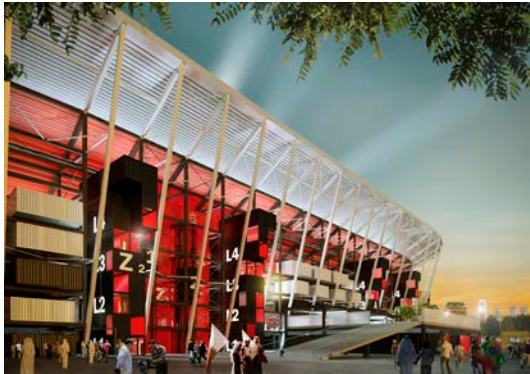
An indirect lighting highlights the prominent color scheme in the twilight © Fenwick Iribarren Architects
