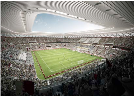
The roof structure is also designed in modules which allows the re-use for other venues. © Fenwick Iribarren Architects
