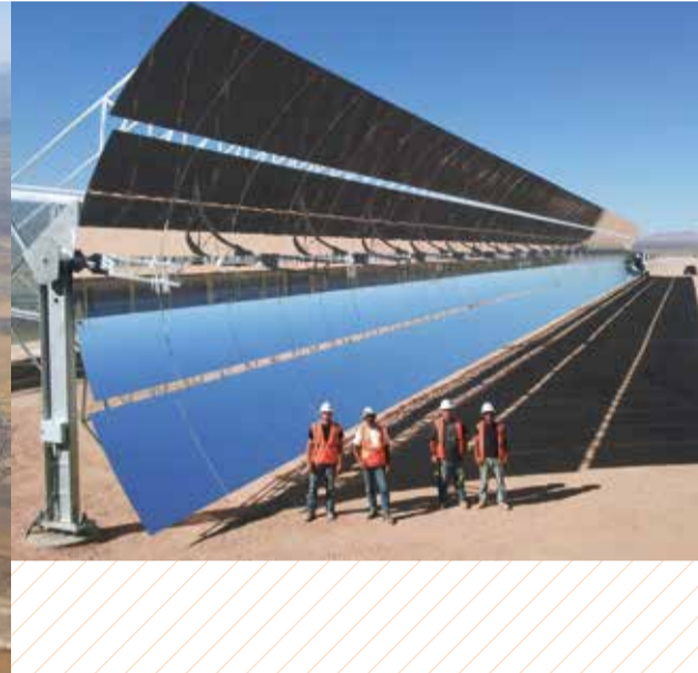
先进的膜吸定日镜 ASM 150, 150 m 2 的聚光面积 Advanced Stressed Membrane heliostat, 150 m 2 concentrator area
